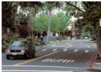
Speed humps and speed bumps force traffic to slow down.
